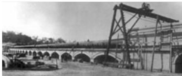
The Western Suburbs sewer viaduct over Cooks River, under construction around 1898.
