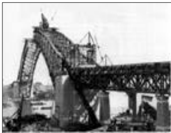
The part completed arches with anchor cables
