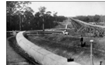
Hudson's temporary scheme, with permanent main under construction
