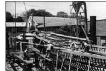
Goat Island shipwrights building pilot vessel 1950s
