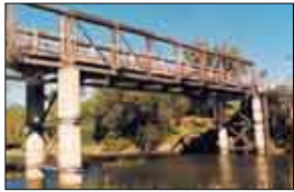
A typical de Burgh truss
