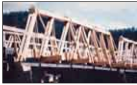
A typical Dare composite truss, at Bulga
