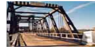
This large 1899 timber truss bridge at Woodville (3) is one of only two overhead braced Allan trusses in service; the other is the nearby Morpeth bridge (1).
